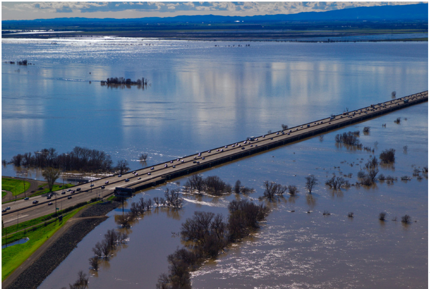
The Yolo Bypass, shown here in use to divert floodwaters away from Sacramento in 2017, is an example of the type of flexible, dynamically managed, multi-benefit water infrastructure that will be increasingly needed as climate change transforms how, when, and where California gets water.
