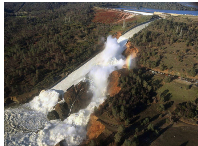
Lake Oroville, California’s second largest reservoir, went from record low levels in 2014 (left) to flood conditions requiring the use of its main and emergency spillways, which failed under the extreme flows, in 2017 (right). Climate projections agree on increases in both extreme drought and extreme flood risk. The state must begin planning and adapting the water system for these future conditions now.
