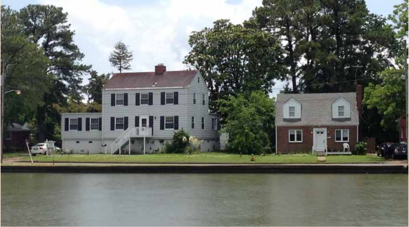
While some residents in Norfolk's frequently flooded Larchmont neighborhood are elevating their homes to avoid flood damage and to lower insurance rates, others either choose not to or cannot afford to.
