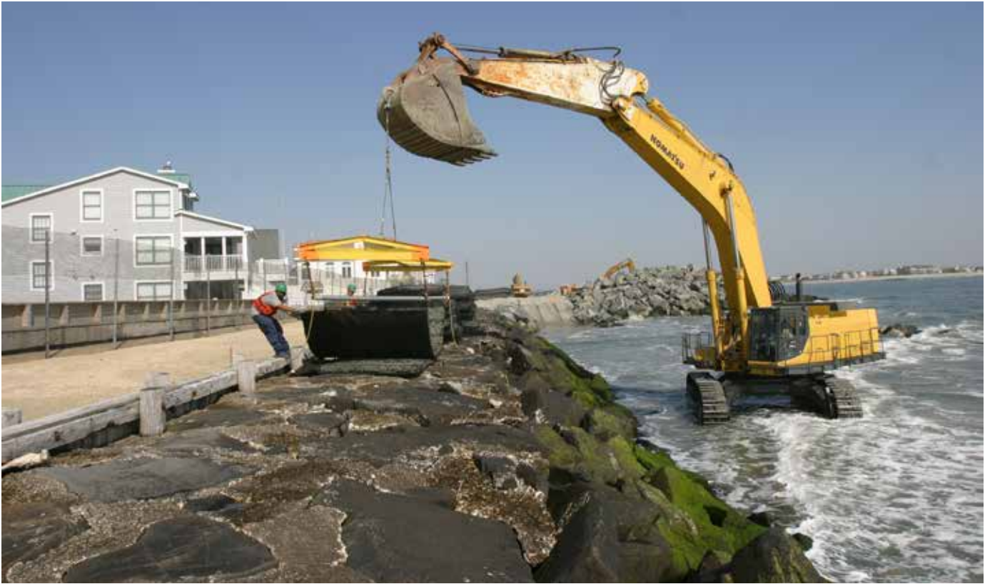
This 2.2-mile-long seawall in New Jersey is part of a project by the U.S. Army Corps of Engineers to protect the shoreline. The project also entails creating 4.3 miles of beach that is 150 feet wide, and replenishing the sand every three years. Whether such projects are sustainable or widely replicable is unclear.
