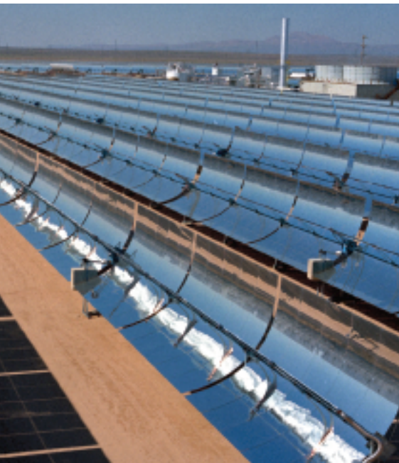
Photo: Warren Gretz, NREL
