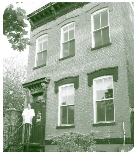
Stephen Young's renovations have made his home more comfortable and energy-efficient.
