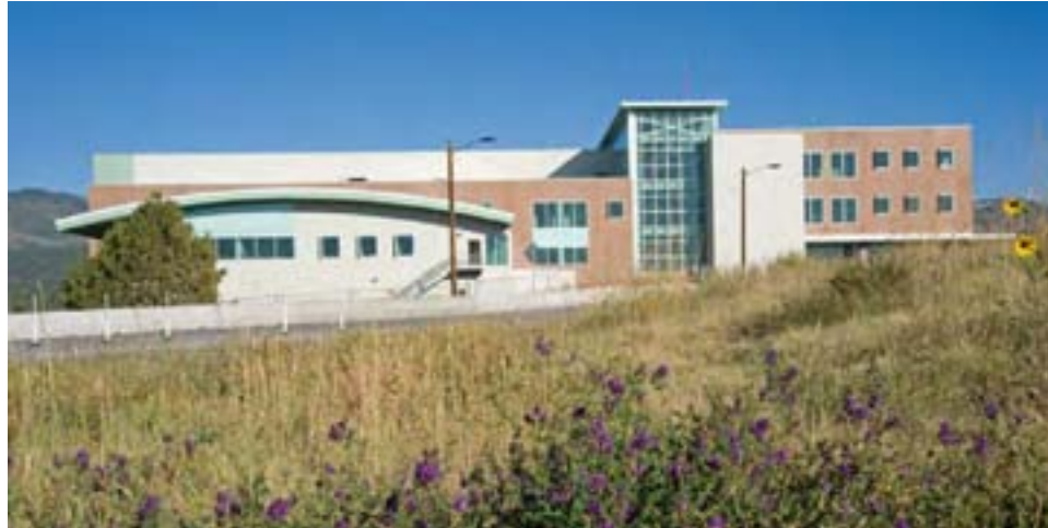
Figure D-9. Chemistry and Metallurgy Research Replacement Radiological Laboratory/Utility/Office Building circa November 2009.
