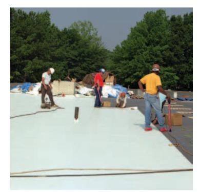
Simple, common-sense decisions often make a significant difference in the long run. Light-colored roofs, like this one at Atlanta's Energy and Environmental Resource Center, reflect sunlight, keeping buildings cooler, reducing demand for air conditioning, lowering electricity use, and saving money.
