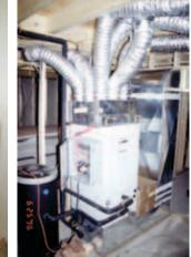
system with centrally located ducts eliminates heat loss.
