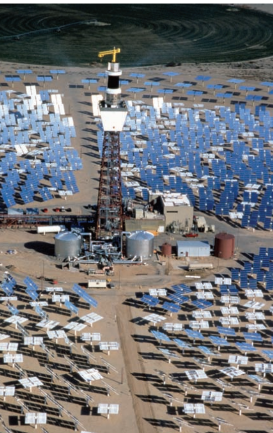
Power towers focus sunlight on a centralized boiler.
