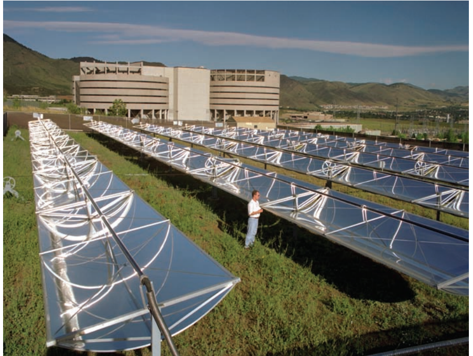
Parabolic troughs produce steam by concentrating sunlight on fluid-filled pipes.
