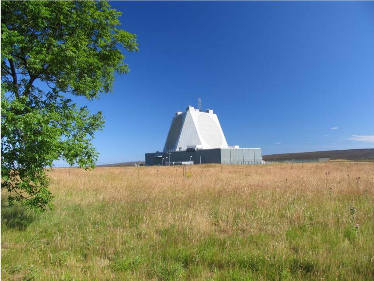
***Fylingdales Upgraded Early Warning Radar (UEWR) at Royal Air Force Station Fylingdales, England. UEWRs form the core of the BMD sensor infrastructure, and are used to track missiles but do not have sufficient resolution to provide discrimination capability.*** Photo: Missile Defense Agency.
