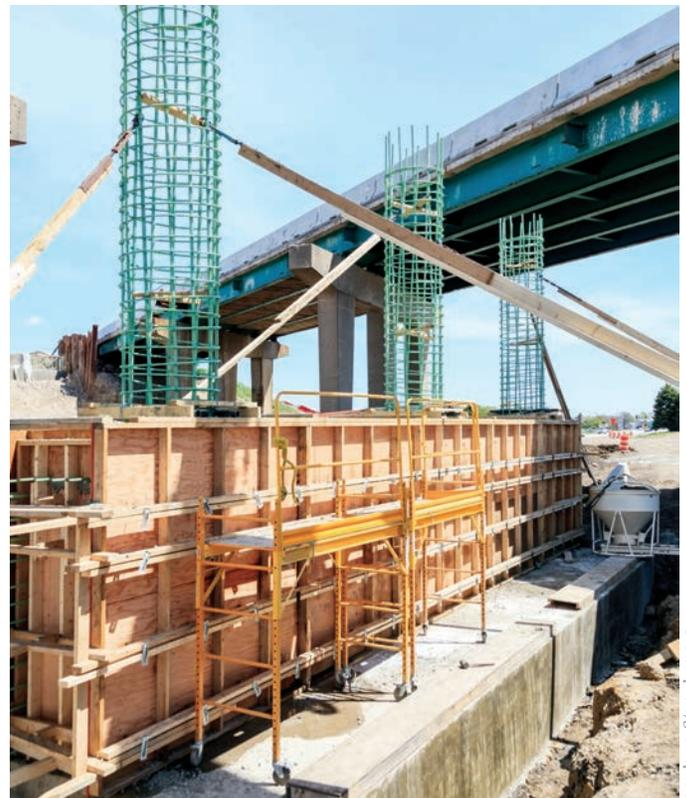
*When concrete is poured for building foundations, workers use plywood or particleboard as a form and then discard it once the cement has hardened.*
