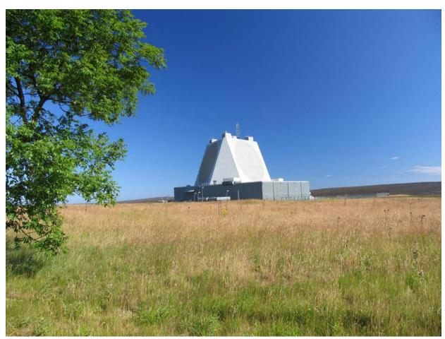
Fylingdales Upgraded Early Warning Radar (UEWR) at Royal Air Force Station Fylingdales, England. UEWRs form the core of the BMD sensor infrastructure, and are used to track missiles but do not have sufficient resolution to provide discrimination capability. Photo: Missile Defense Agency.
