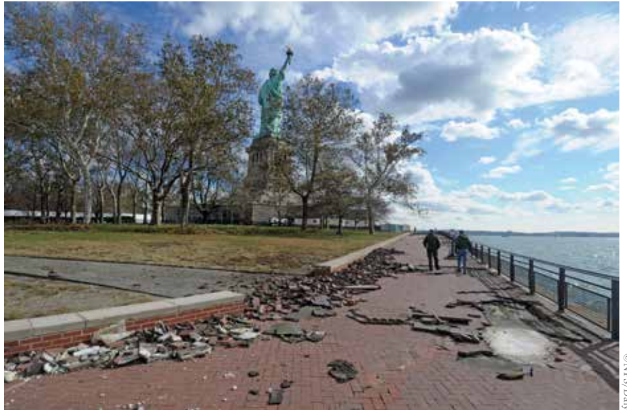
Hurricane Sandy's massive storm surge destroyed most of the radio equipment, electrical infrastructure, and security systems of both Liberty and Ellis Islands. Floodwaters inundated three-quarters of Liberty Island—some of the aftermath is pictured—and the beloved landmark was closed to the public for more than eight months.
