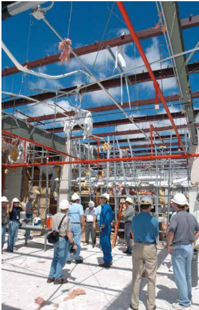
This building at Kennedy Space Center was almost totally unserviceable after losing approximately 35 percent of its roof to Hurricane Frances in 2004.
