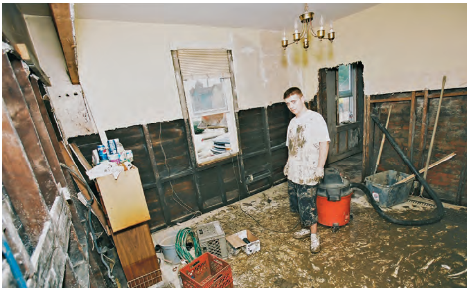
After a 2004 flood inundated this home in Bridgeville, PA, its baseboard and insulation were removed to prevent mold and mildew, which may trigger respiratory illnesses. Floodwaters can pose additional health risks if they become contaminated with chemical pollutants, agricultural runoff, or raw sewage. Even after the water has receded, residents often struggle with stress and other mental health problems.
